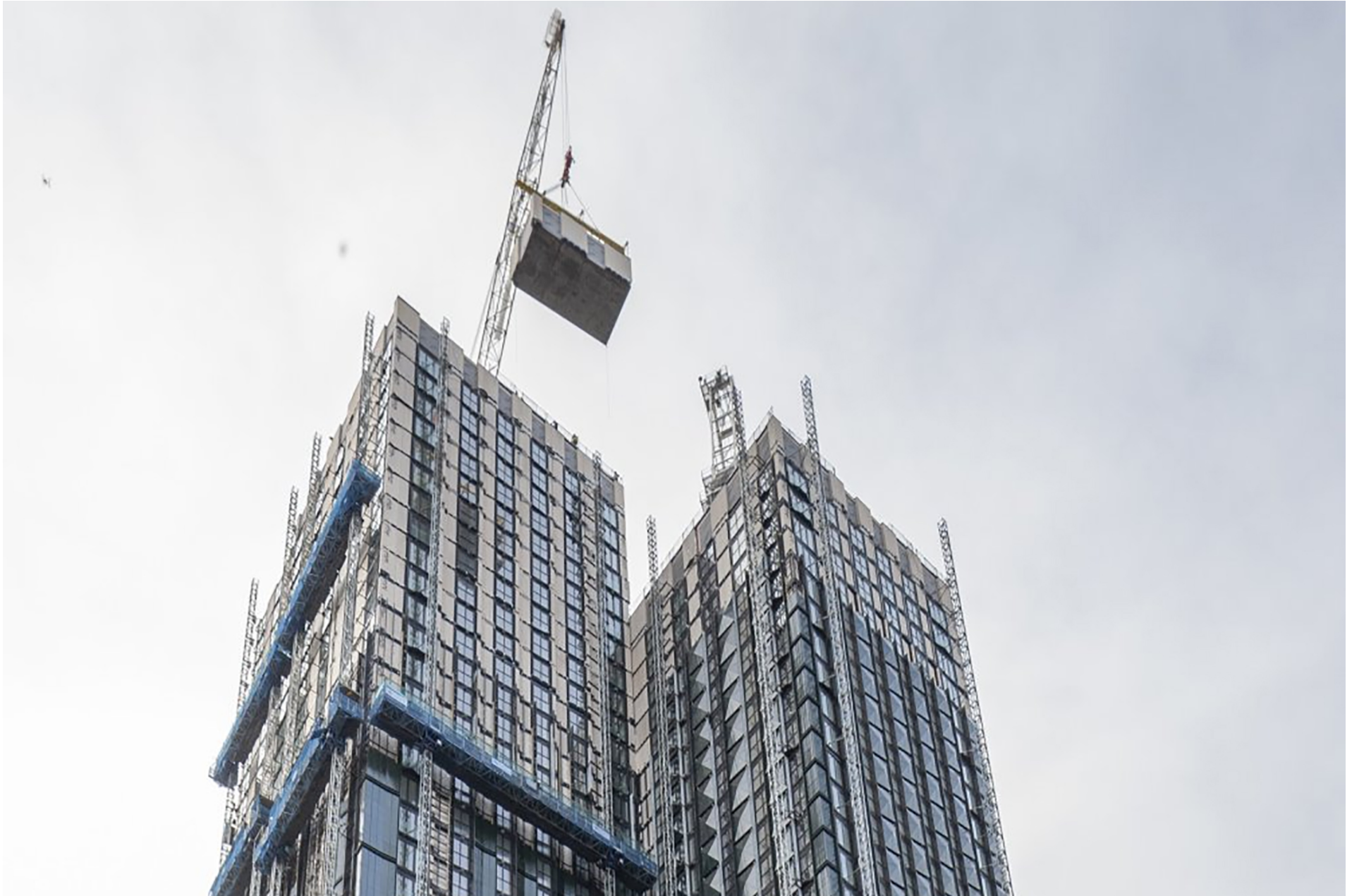
A crane lifts the final module on a London residential building that's expected to be the world's largest modular tower. (HTA Design)
